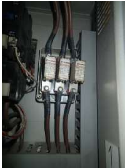
All controller main fuses must be correctly installed and covered
