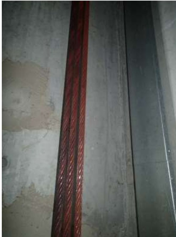
Rusty hoisting ropes must be replaced
