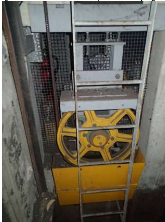
Traction sheave guards must be correctly installed
