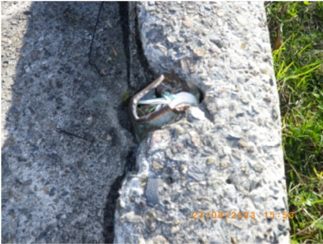
SP52948 unprotected electrical cables Block A basement creating OH&S risk for many years
