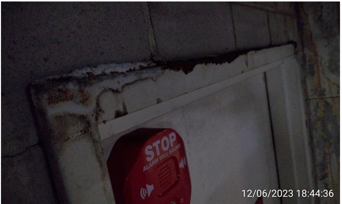
—SP52948-Block-A-basement-external-fire-door-2-rusted-for-seven-years-due-to-water-leaks-photo-1-11jun2023.webp
