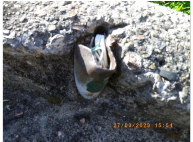
SP52948 unprotected electrical cables Block A basement creating OH&S risk for many years
