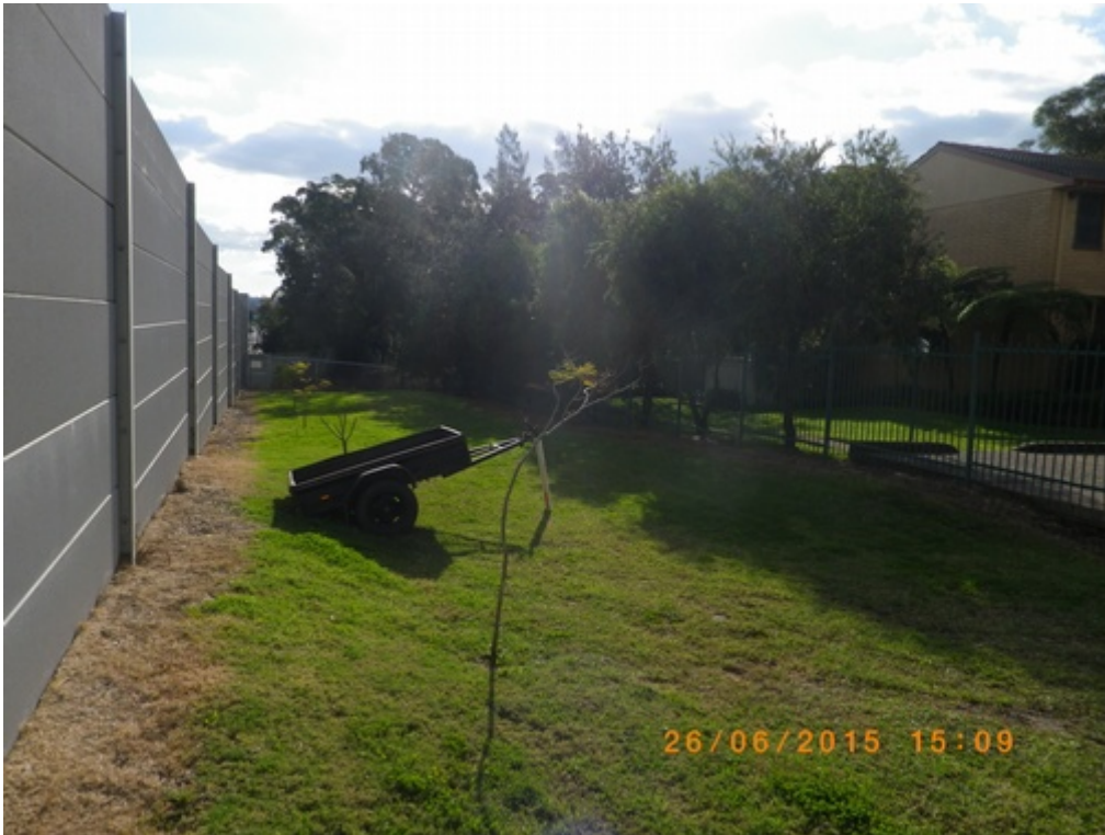
Owners corporation maintenance staff allowing unauthorised parking on council land towards M2 motorway noise barrier on 26 th of June 2015
