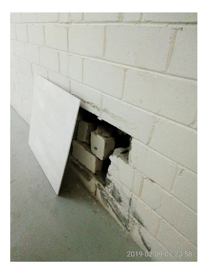
SP52948 Block C Level 6 large hole in wall simply riveted by large panel and no further repairs occurred on  $16^{th}$  of February 2019
