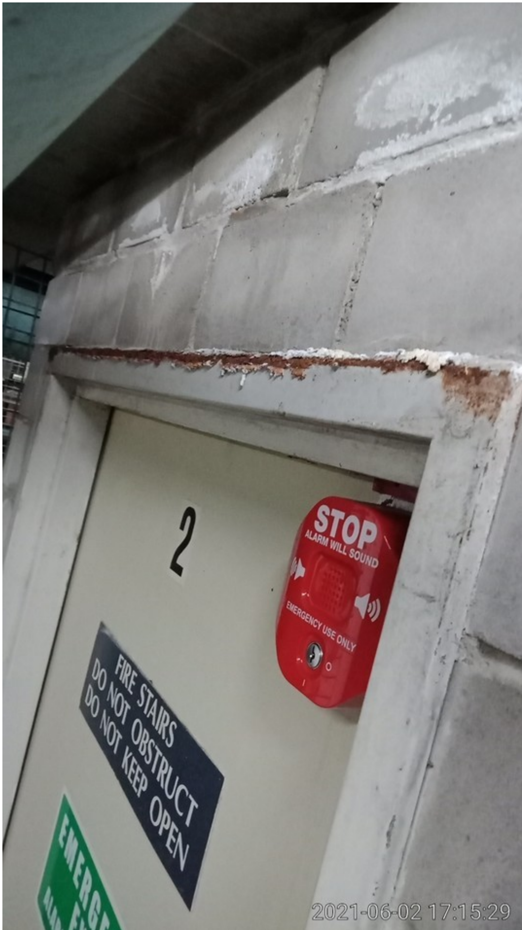
24 Rusted frame of fire door for six years – Block A basement
