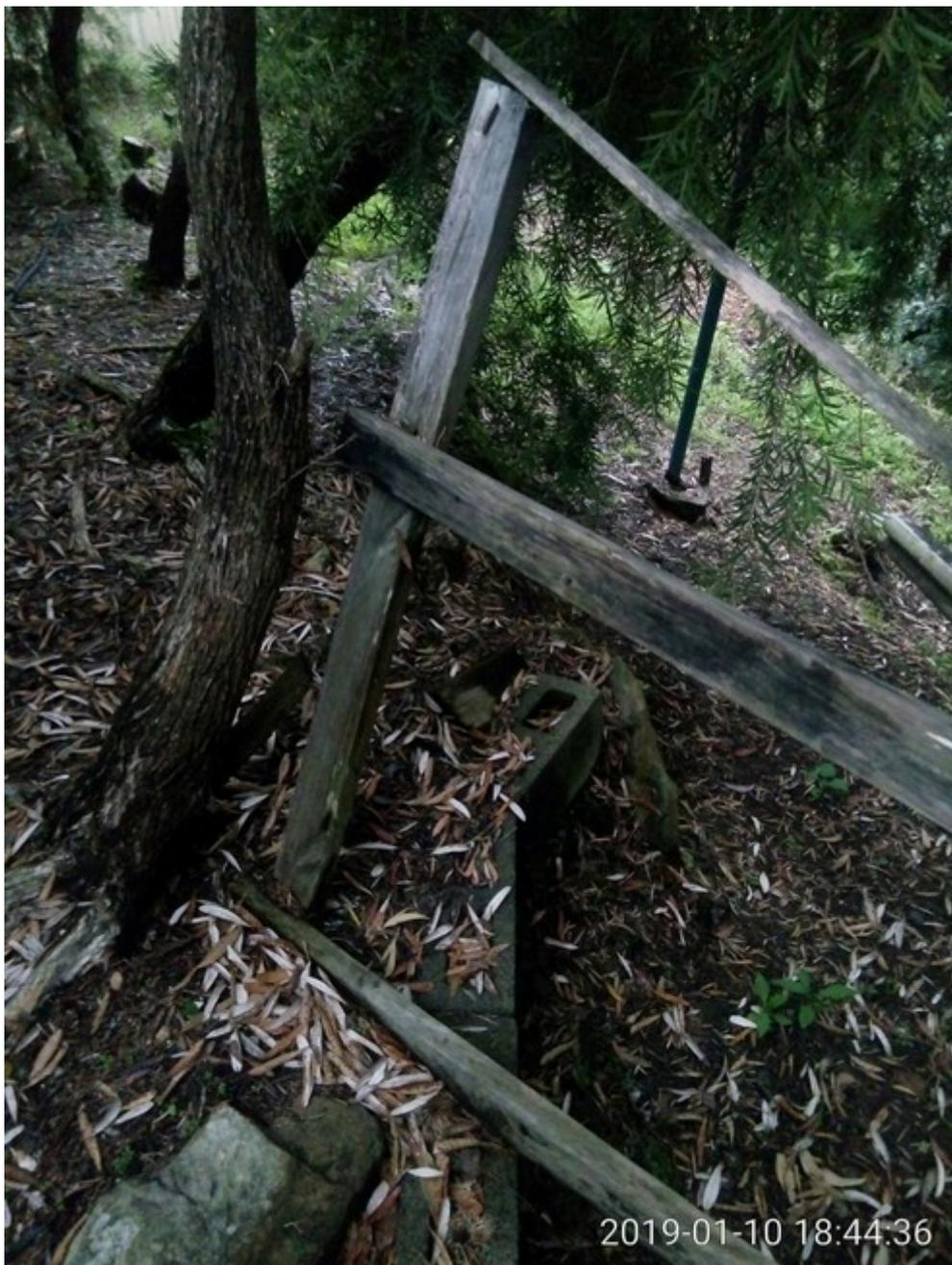
SP52948 - Collapsed wooden railings behind townhouses on 19<sup>th</sup> of January 2019
