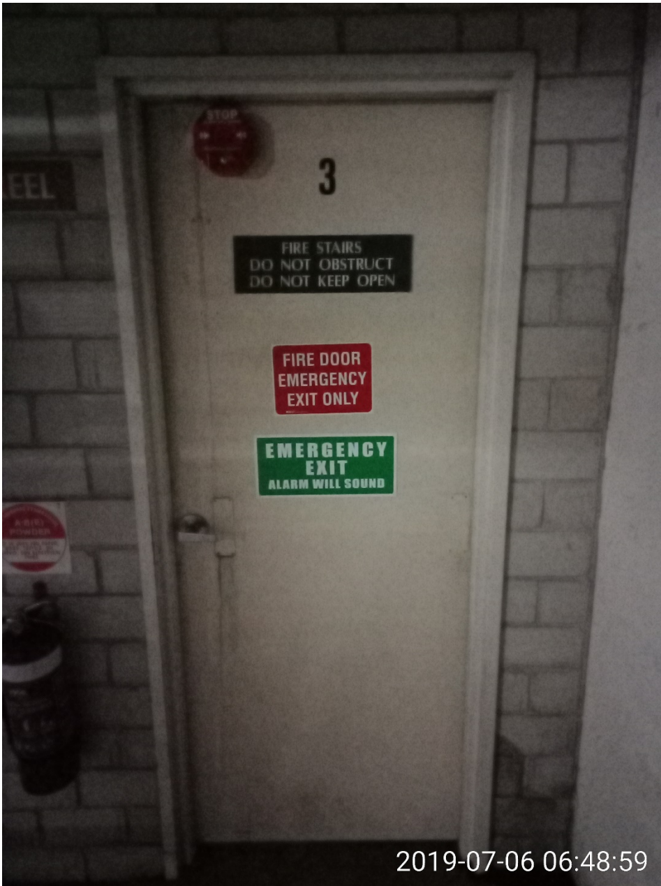
Fire door 3 (final exit door)
