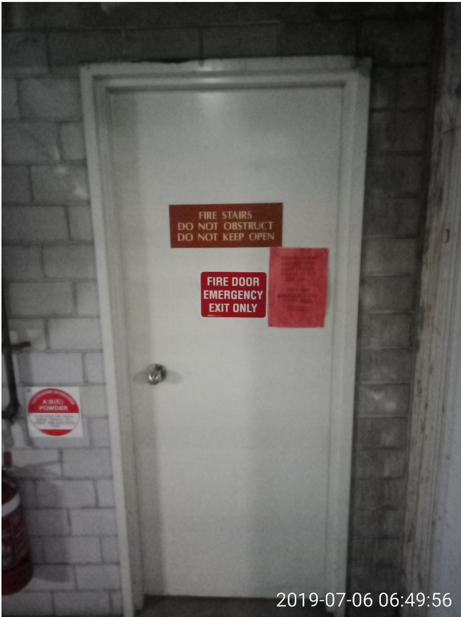
Fire doors 4 (internal going towards fire stairs and final exit door)
