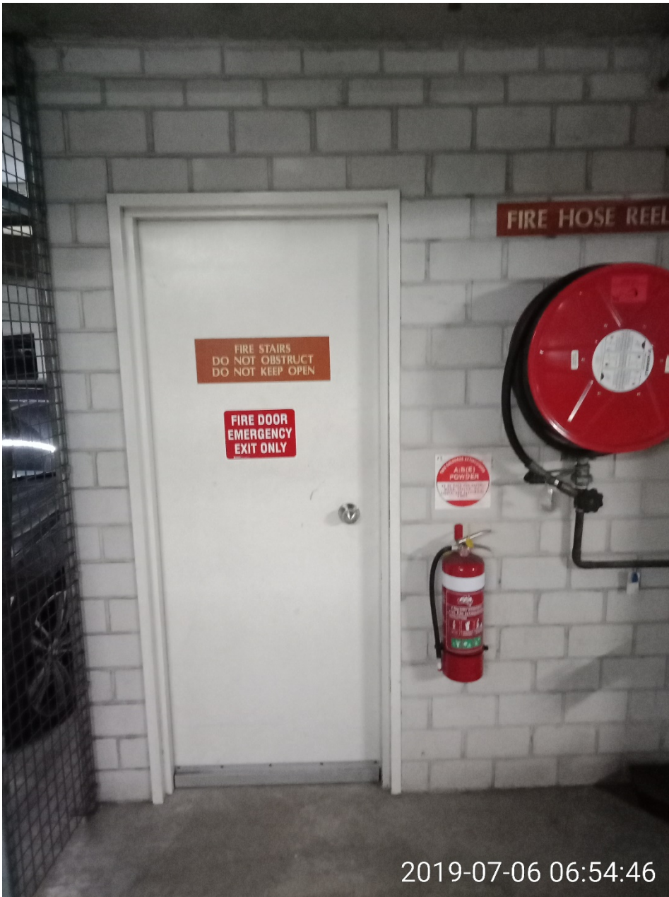
Fire doors 7 (internal going towards fire stairs and final exit door)
