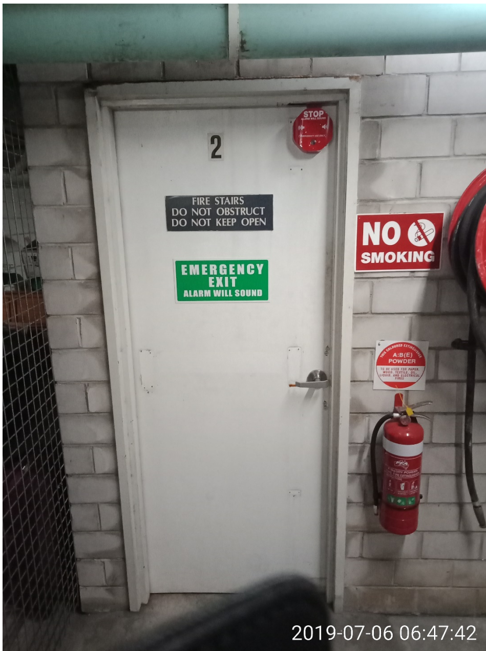
Fire door 2 (final exit door)
