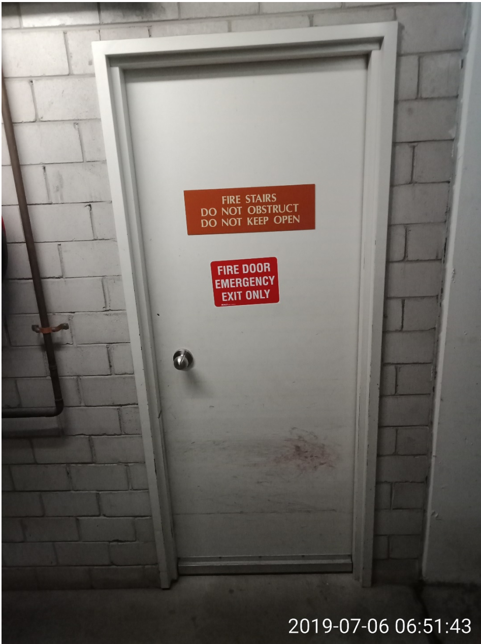
Fire doors 5 (internal going towards fire stairs and final exit door)
