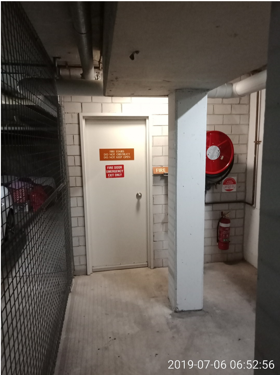
Fire doors 6 (internal going towards fire stairs and final exit door)
