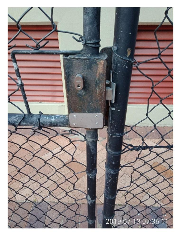
SP52948- Rusted lock on tennis court - paint after second owner's complaint about incomplete repair -  $11^{th}$  of August 2019
