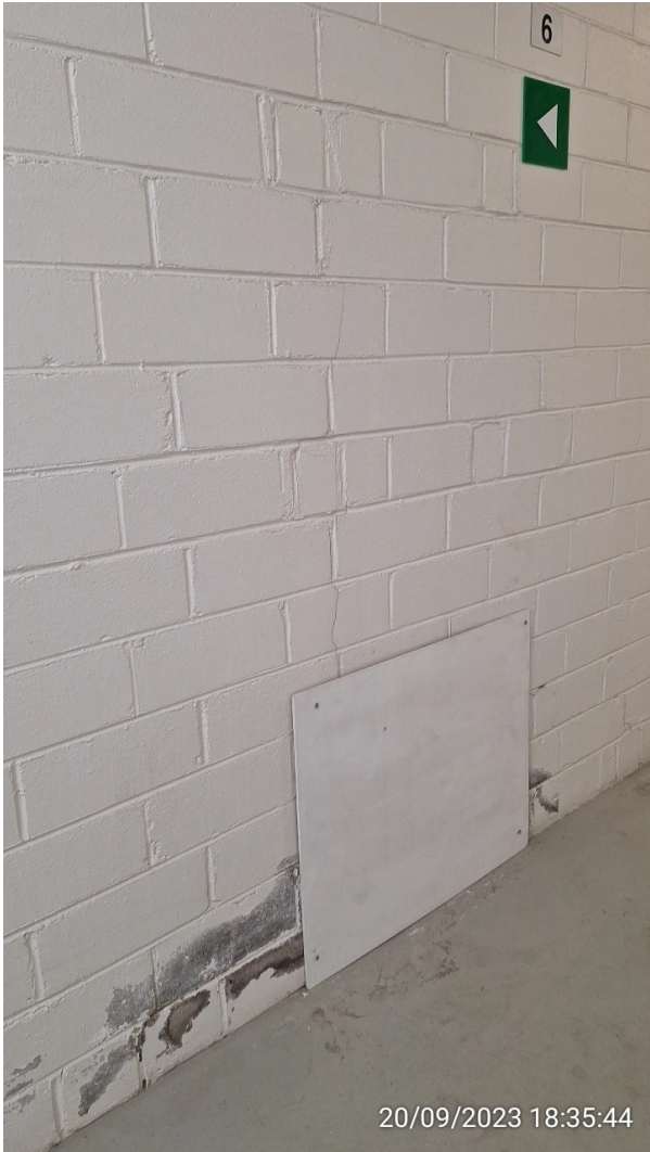
Block C level 6 fire stairs – unrepaired wall due to water leaks since February 2019, and Block C ground floor fire exit – unrepaired wall due to water leaks since June 2021
