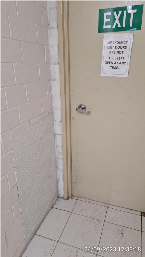
Block C level 6 fire stairs – unrepaired wall due to water leaks since February 2019, and Block C ground floor fire exit – unrepaired wall due to water leaks since June 2021
