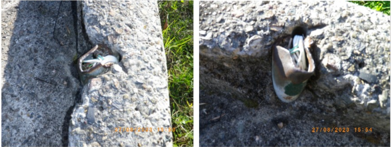
SP52948 unprotected electrical cables Block A basement creating OH&S risk for many years
