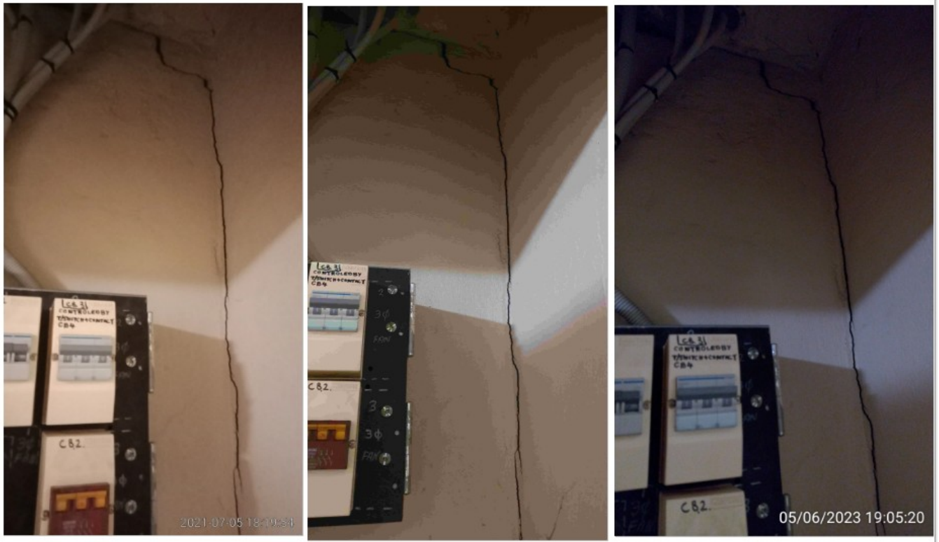
SP52948-Block-B-level-7-neglected-large-wall-crack-telecom-and-electrical-cabinet-5Jun2023.png
