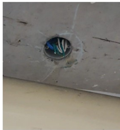
SP52948 unprotected electrical cables Block A basement creating OH&S risk for many years
