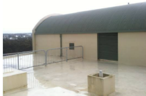
Block C roof coverings
