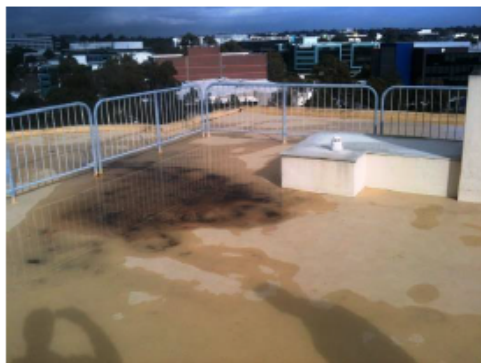
Block A roof coverings
