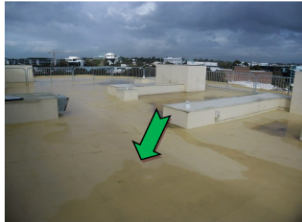
Photo 2. Block A, roof, floor – non-asbestos textured coating
