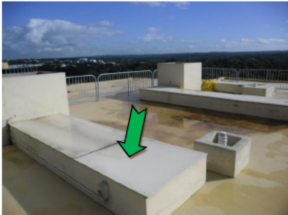
Photo 1. Block A, roof, box covers – non-asbestos containing compressed fibre cement panels
