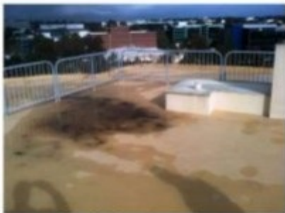
Block A roof coverings
