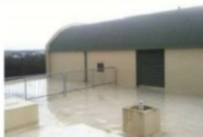
Block C roof coverings
