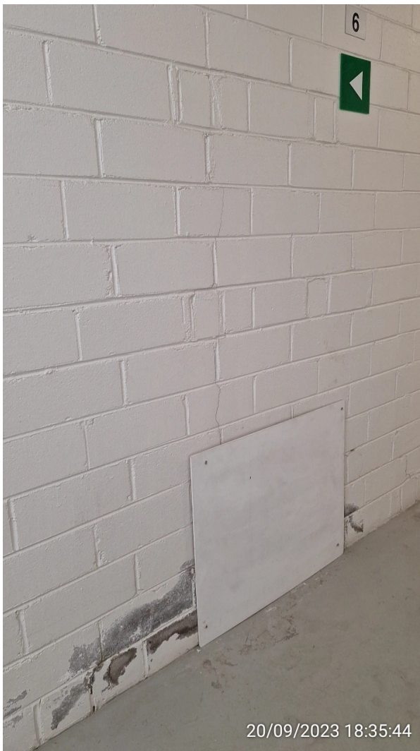
Block C level 6 fire stairs – unrepaired wall due to water leaks since February 2019, and Block C ground floor fire exit – unrepaired wall due to water leaks since June 2021
