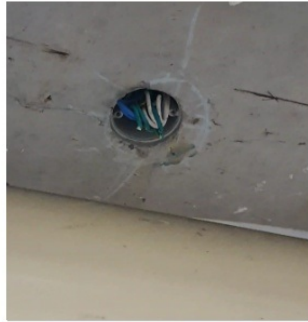
SP52948 unprotected electrical cables Block A basement creating OH&S risk for many years
