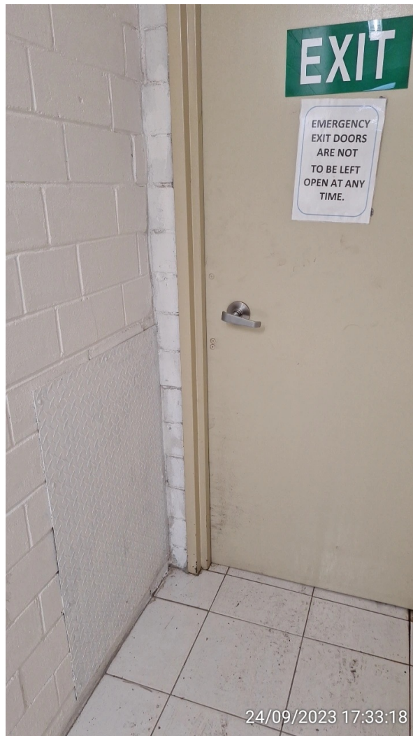
Block C level 6 fire stairs – unrepaired wall due to water leaks since February 2019, and Block C ground floor fire exit – unrepaired wall due to water leaks since June 2021
