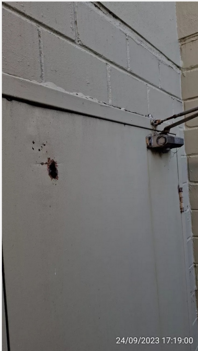
7. Examples of burnt external fire door in Block A, photographed on 24 September 2023 and 23 October 2023:
