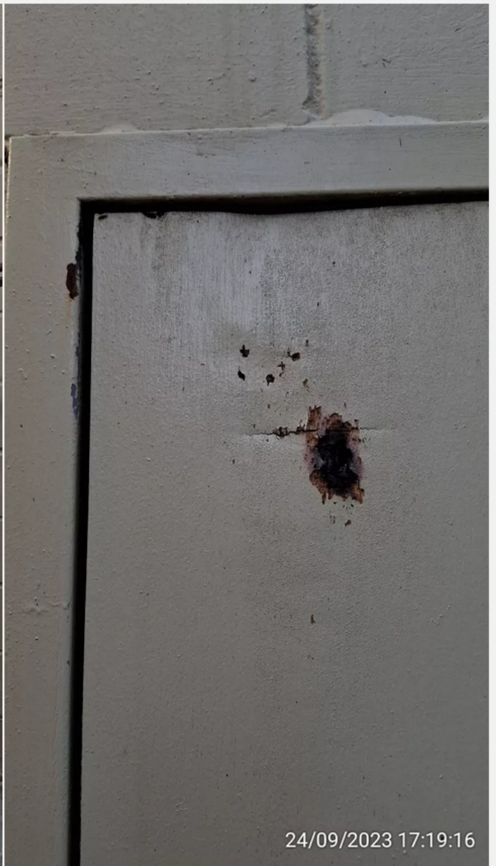
7. Examples of burnt external fire door in Block A, photographed on 24 September 2023 and 23 October 2023:
