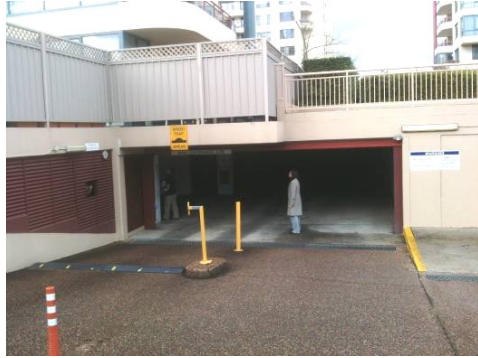
Car park entry
