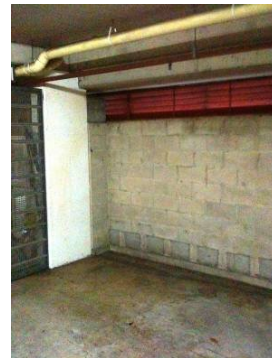
Internal car park ramp
