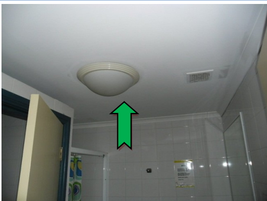
Photo 5. Spa facilities, change rooms, ceiling – non-asbestos fibre cement sheeting
