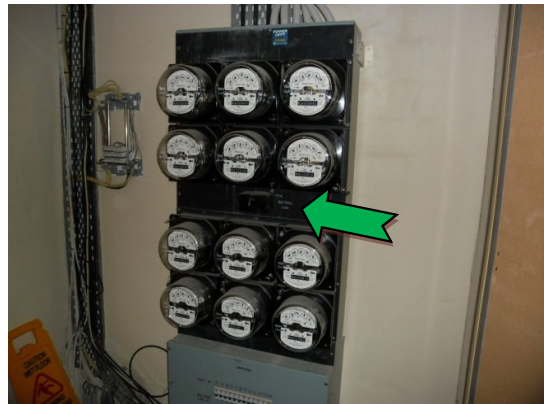
Photo 4. Electrical boards, throughout Block A, B, C & D – non-asbestos bakelite panels
