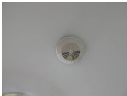
Typical domestic type smoke detector
