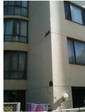
Isolated patch repair awaiting redecoration
