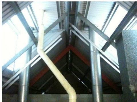
Steel structure to plant room
