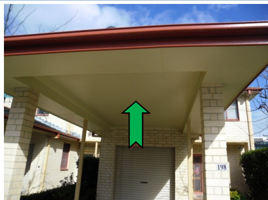
Photo 6. Terrace houses, carport awning – non-asbestos fibre cement sheeting
