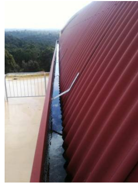
Block A ancillary roof gutter
