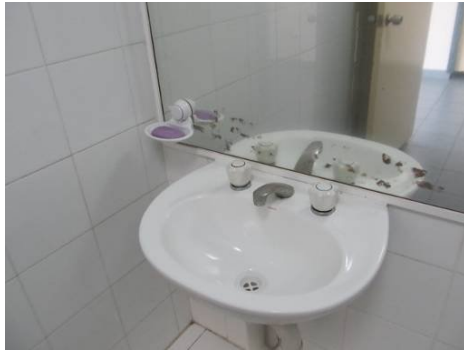
Typical vanity basins
