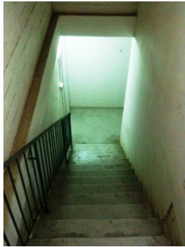
Typical view of fire stairs
