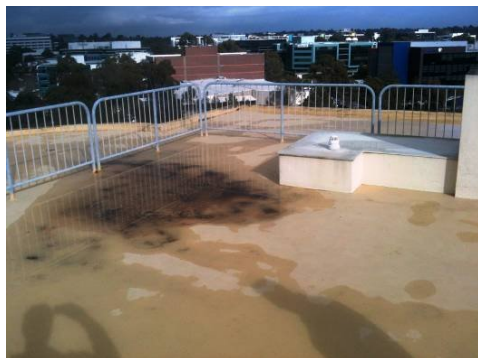
Block A roof coverings
