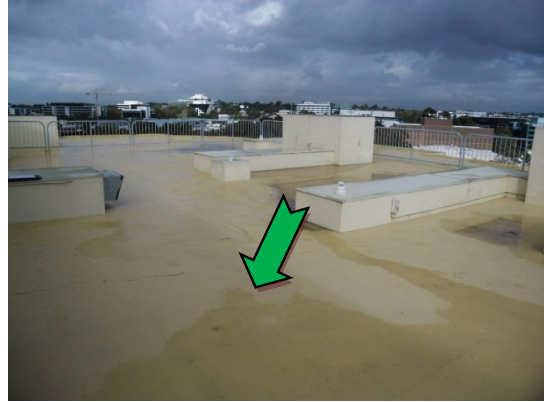
Photo 2. Block A, roof, floor – non-asbestos textured coating
