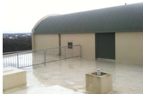
Block C roof coverings
