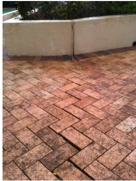
Isolated raised paving
