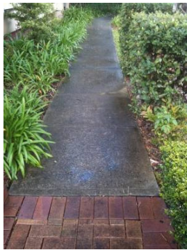
Brick paving and concrete footpaths
