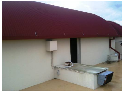
Block A ancillary roof
