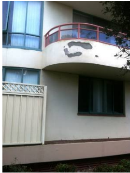
Isolated patch repair awaiting redecoration
