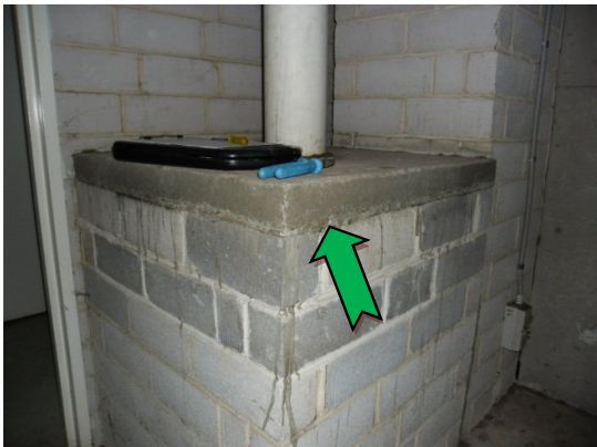
Photo 3. Block A, roof, plant room, packer – non-asbestos compressed fibre cement panel
