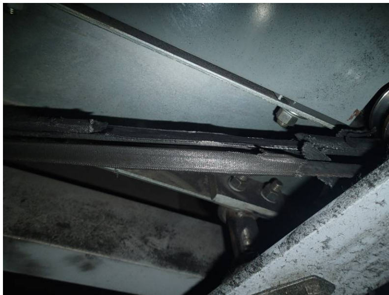
Worn power door operator drive belts must be replaced before they fail
